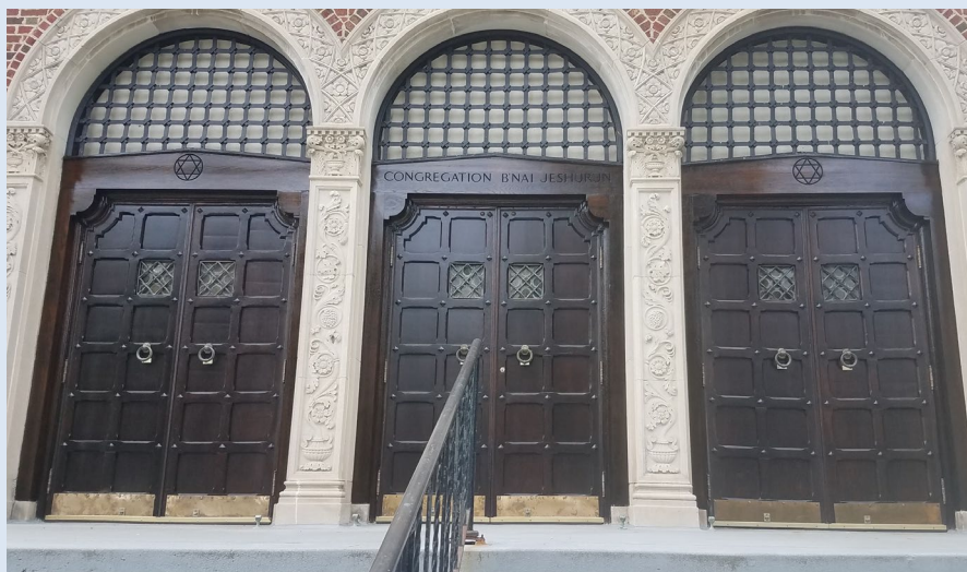
Here is the finished set of doors! Ready for another 96 years of Nebraska weather...
